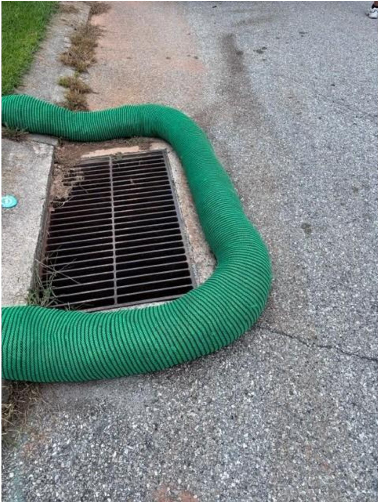
MS4 storm water preventive maintenance
