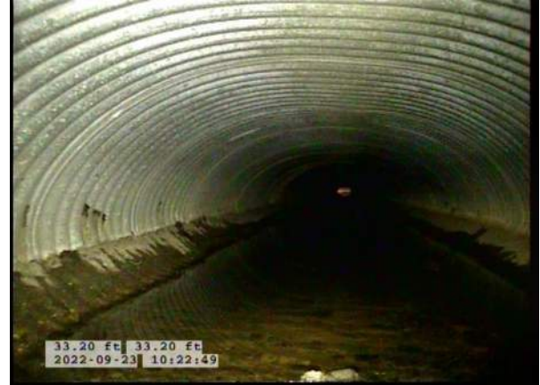
6, 00:02:14, 33.20ft Water Level, 10% of the vertical dimension
