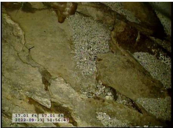
7, 00:01:53, 16.23ft Surface Damage Missing Wall from 5 o'clock to 7 o'clock / BOTTOM OF PIPE RUSTING AWAY
