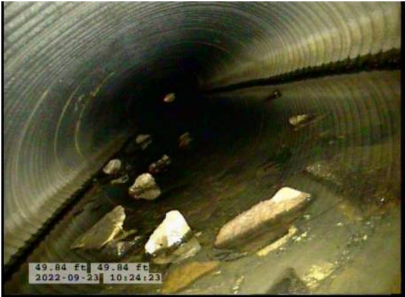
9, 00:03:24, 49.84ft Deposits Settled Compacted, 10% of cross sectional area from 5 o'clock to 7 o'clock, within 8 inch, Start
